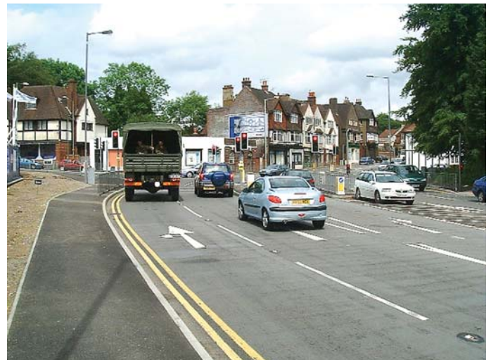
The MOVA junction on the A3 at Hindhead
