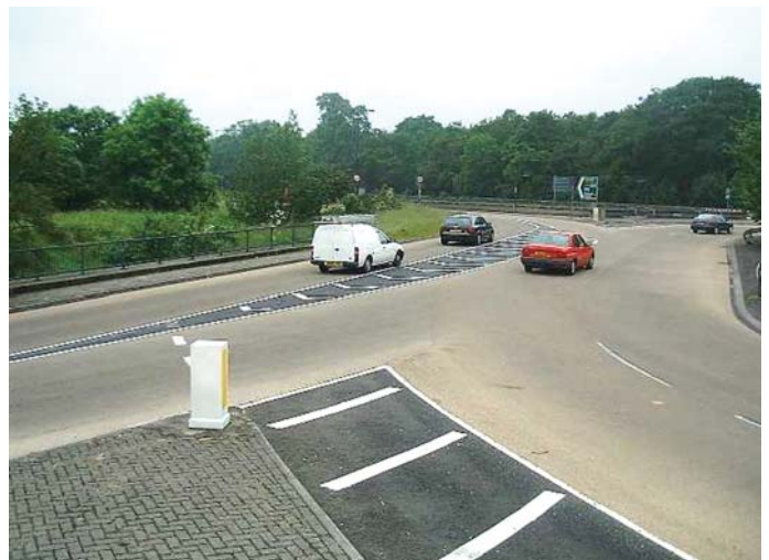
A view of the free left turn lane at the Wimbledon Park Side entry
