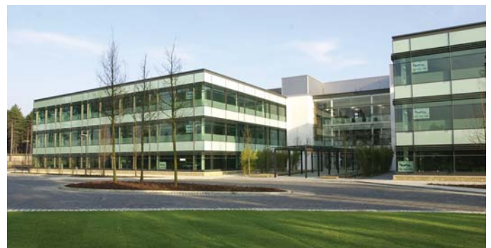
TRL's brand new offices in Crowthorne
