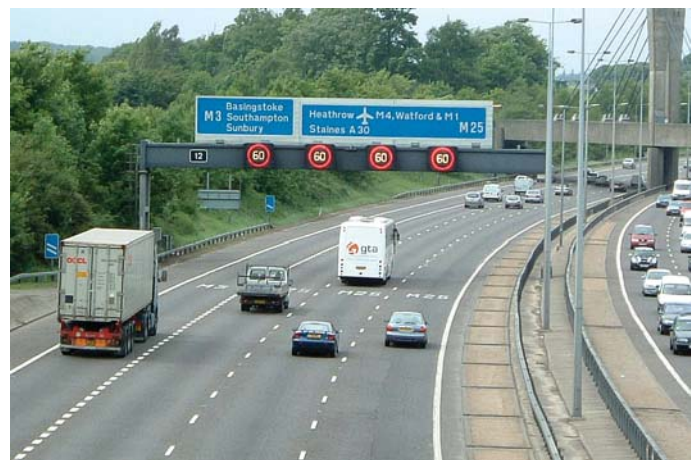
An M25 MIDAS system signal gantry
